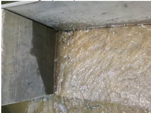
Photo of water leaking through weir.
