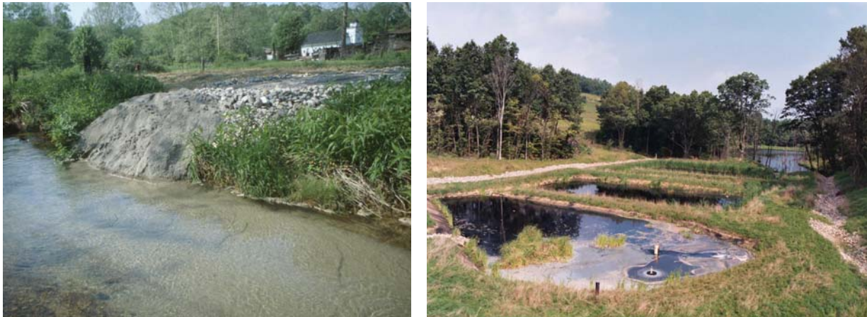
Figure 1. Strategic treatment of AMD by a suite of methods such as active lime sand dosing operation (left) or passive treatment wetlands (right), demands tools for performance measurement.
